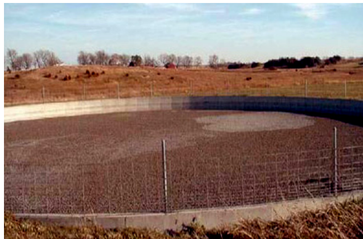
Figure 5.2 Lightweight expanded clay aggregate (LECA) cover on a concrete manure storage tank
