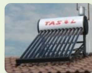
Example of a solar water heater installed by the PoA. Photo: SASSA PoA Design Document
